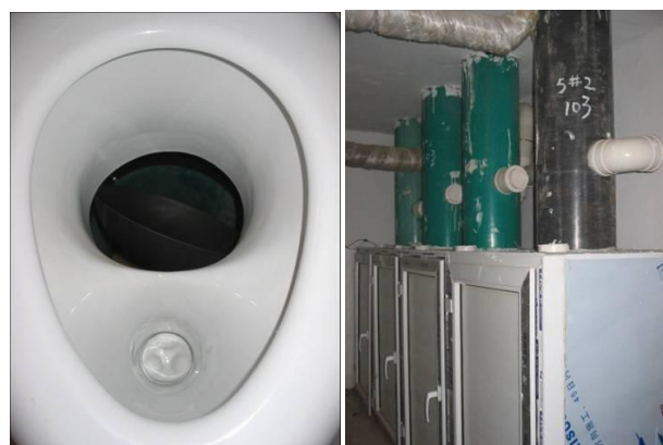
Figure 16. Left: Ceramic urine diverting dry toilet equipped with faeces turning bowl and odour trap for urine. Right: Downpipes coming from each floor leading into separate bins with housing (Erdos Eco-Town, Dong Sheng, China; source: Berger, 2009)
