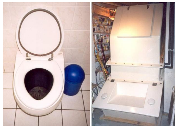
Figure 7. Left: Dry toilet with removable insert and sealed toilet seat. Right: Insulated single-vault composting container with upper lid for maintenance and lower lid for discharge and working platform (both Hamburg-Allermöhe, Germany; source: Berger and Lorenz-Ladener, 2008).
