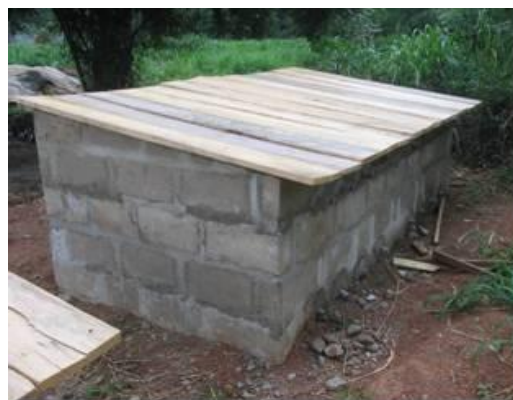
Figure 2. Brick chamber for faeces composting equipped with vent pipes on the back side and sheltered (at German Research project at Valley View University, Ghana; source: Berger, 2009)
