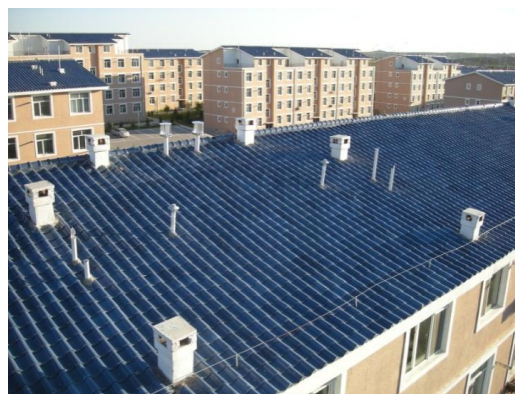
Figure 15. Part view of the multi-story houses in Dong Sheng, showing vent pipes on the roof from the ventilation system (photo: Berger, 2009).
